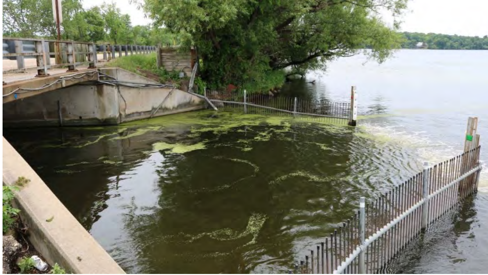
Figure 2-3: Bubble barrier at CTH A bridge where Silver Creek Estuary enters Green Lake. Bubbles block fish entrance during carp spawning season, May-July. Photo taken by Stephanie Prellwitz.
