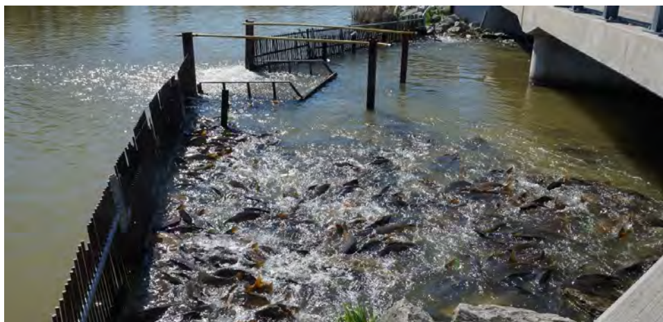
Figure 3-4: The barrier at the CTH K bridge at the outlet of CKM keep carp out of the shallow marsh during spawning season. Photo taken May 5, 2016 by Stephanie Prellwitz.
